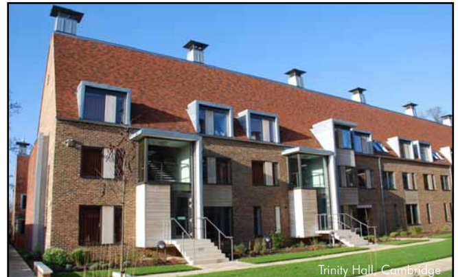
Figure 45: Well defined entrances, projections and ventilation stacks create vertical rhythm. Source: RH Partnership.
